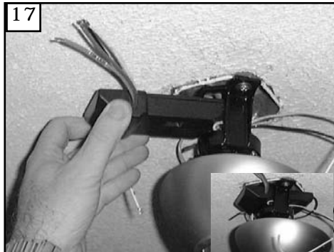
17 Install remote receiver by sliding into opening in the Mounting bracket. Make sure that the dip switches on the Transmitter and the Receiver are set to the same position. See Fig 34 for remote operation
